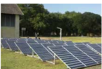
PANEL BEING MOUNTED IN A SCHOOL PLAY GROUND
